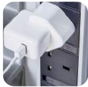
Device adapters plug into 2x8-way powerstrips.
