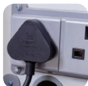
Device adaptors plug into 4x5-way power strips.
